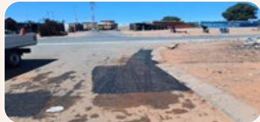
Pothole repaired in October 2024
